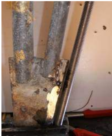
2): Threaded rod before covering with pipe
