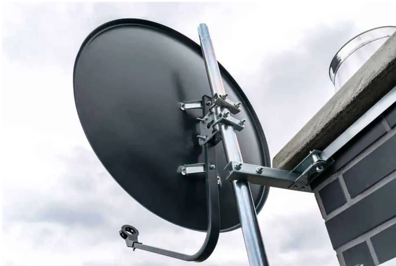
Chimney holder for mounting Starlink antenna
