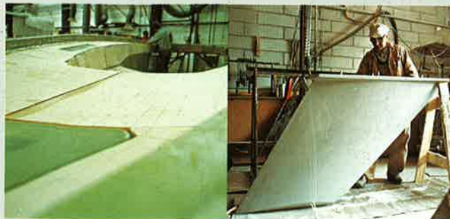
Full sandwich construction on all horizontal surfaces. The keel – an alloy of iron and lead cast in glassfibre. Something else you don’t see every day...
